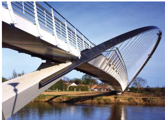
Figure 2. Arch bridge in York, England.
