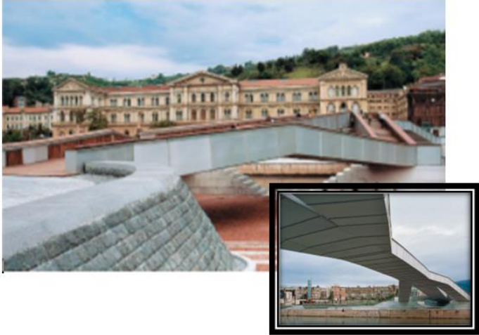
Figure 3. Through bridge in Bilbao, Spain.
