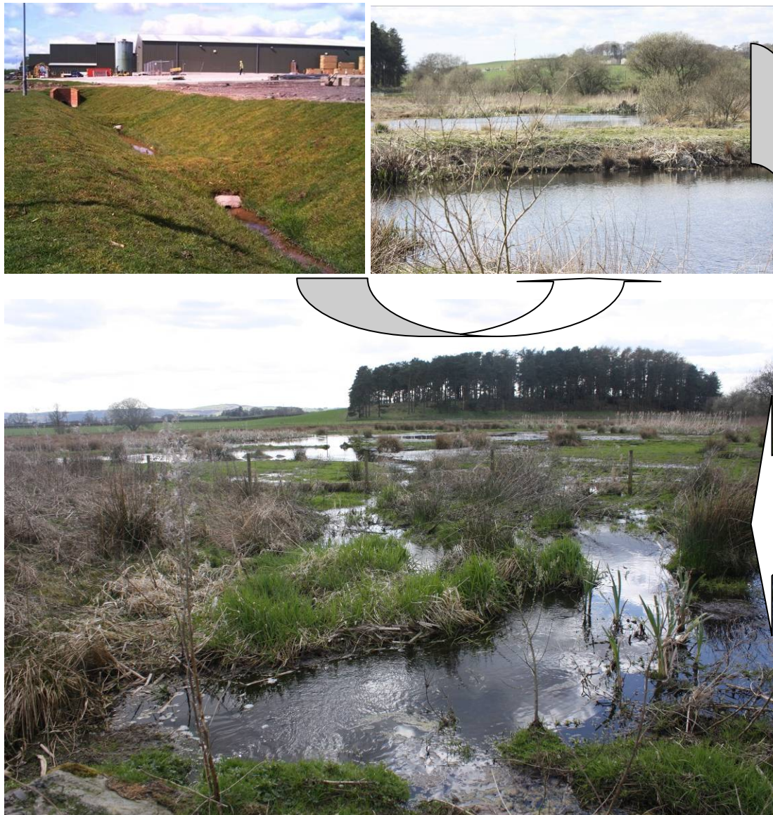
Figure 6.4 The SUDS treatment train at Steven's Croft industrial estate, Lockerbie, showing one of the swales serving units close to source, followed by the two ponds and then the final series of stormwater wetland pools prior to discharge to the watercourse.
