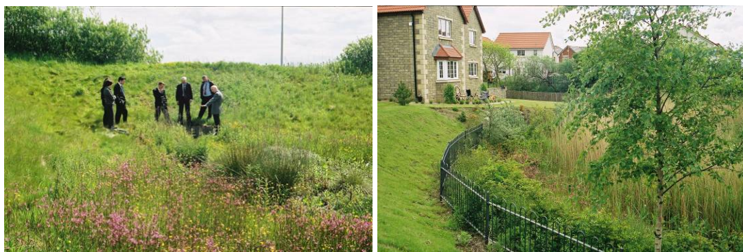
Figure 6.5 Uncut vegetation at a detention basin and a retention pond, Dunfermline.
