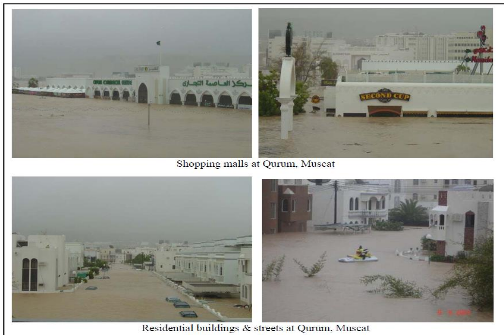
Figure 4.9: Heavy Rain Flooded Urban Streets and Buildings in Muscat
