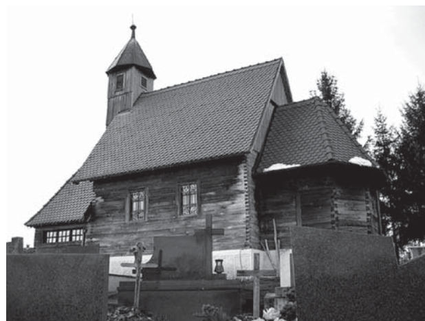
5. Stari Brod, kapela sv. Martina (snimljena 2006., sada u obnovi). / Stari Brod, Chapel of St Martin (photographed 2006, currently in restoration)
