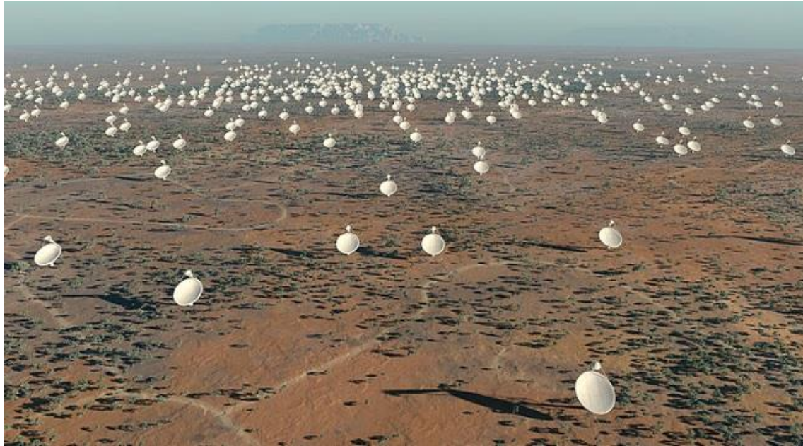
Figure 1 - An artist vision of the SKA Core site, with some of the projected 3000 15-meter parabolic dishes. From http://www.skatelescope.org .
