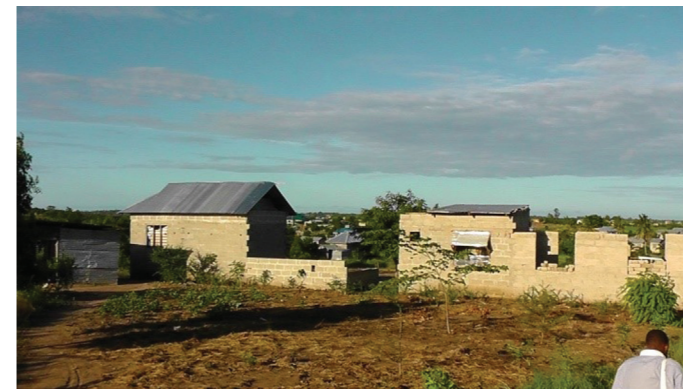
Fig. 4g): Fully built house source: author
