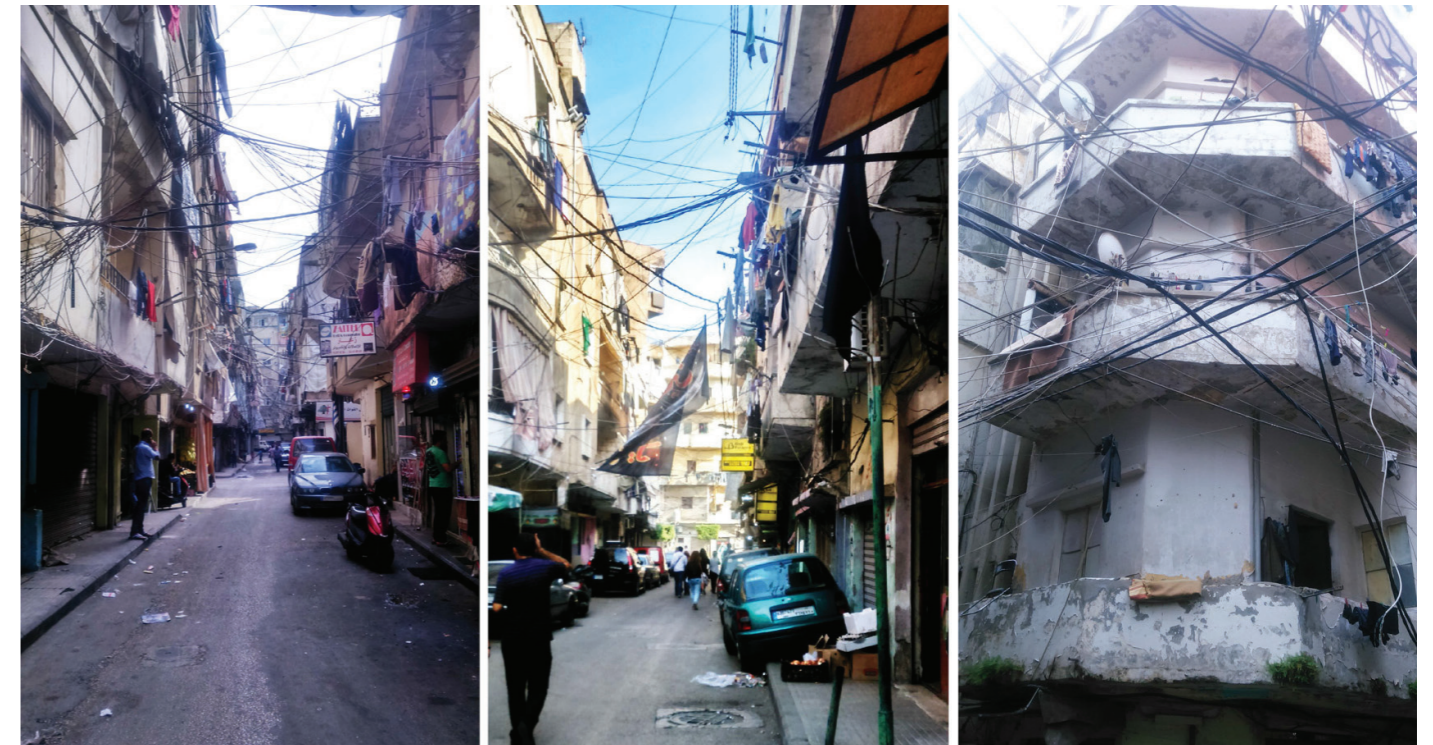
Figure 8: The current conditions of streets, sidewalks and buildings in Nabaa.
