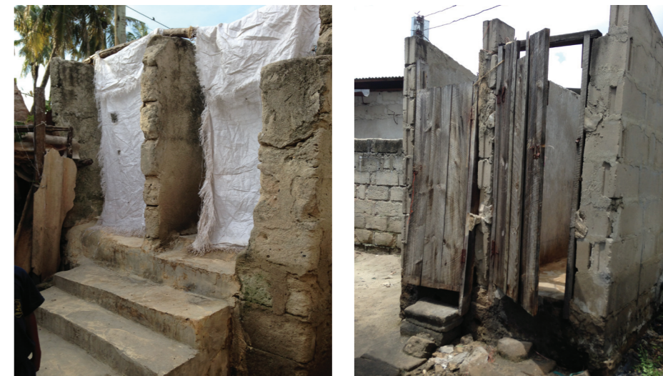
Structural conditions of the toilets in the settlement without doors. Source: Author
