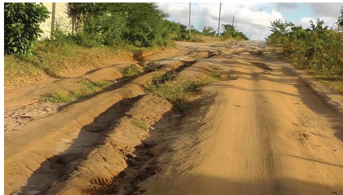
Fig. 4a): Access road to Mabwepande resettlement area source: author
