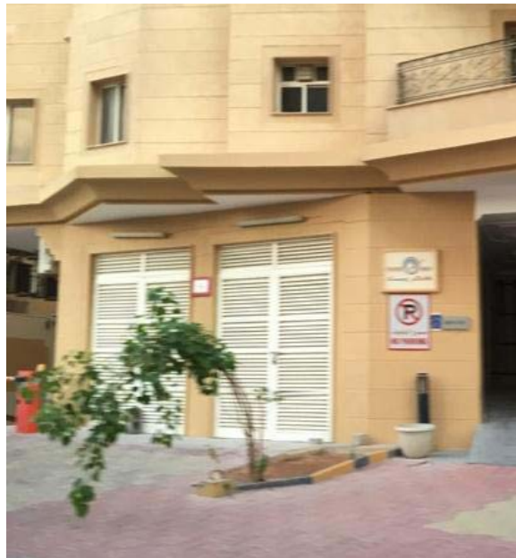
Figure 15. Plant in Al Saad area
