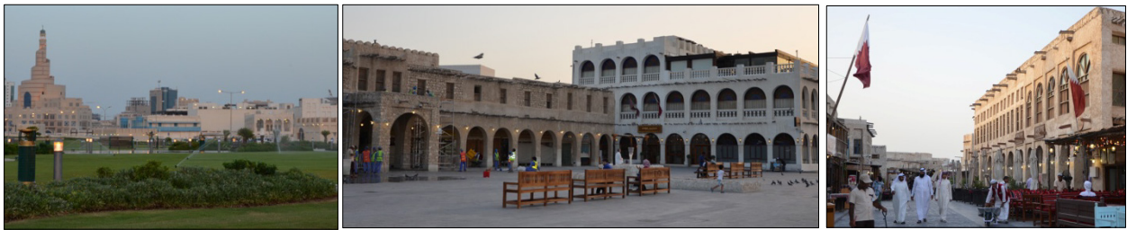
Figure 1-2-3. Views of the Souq Waqif (Photos from the authors)
