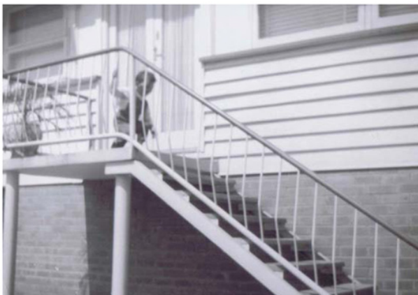
Figure 19. Renovated house. In 1970 Salvatore and Maria purchased a single storey weatherboard house standing on timber stumps in New Farm. In 1971 the house was lifted and the ground floor was enclosed with a brick veneer wall. (Photo from case 2)
