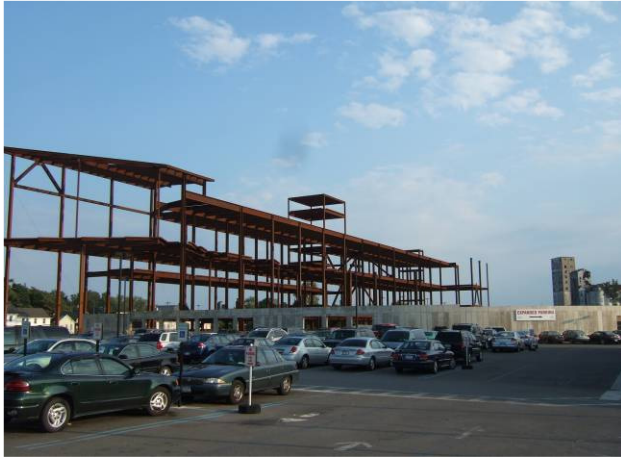
Construction of the new parking ramp at the Buffalo Creek Casino
