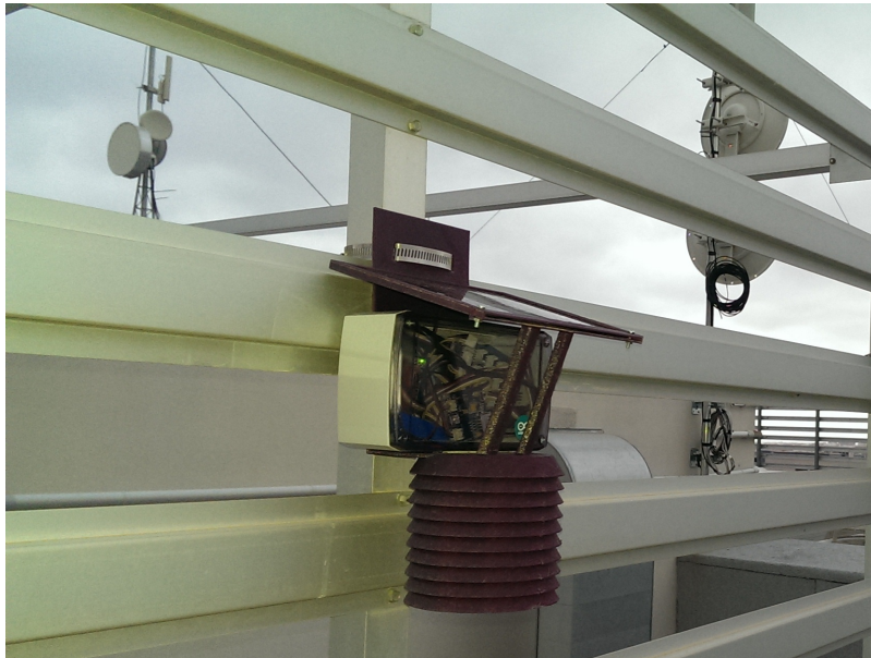
Figure 7: Example of SEnviro Thing installed in Españec 2 building.
