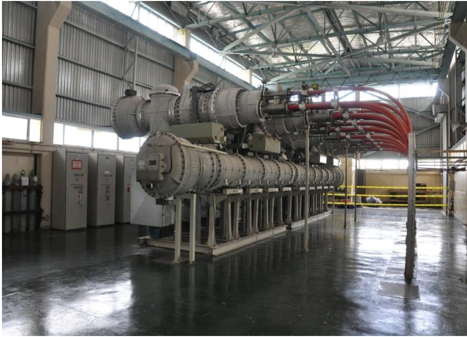
Figure 1. High voltage switchgears
