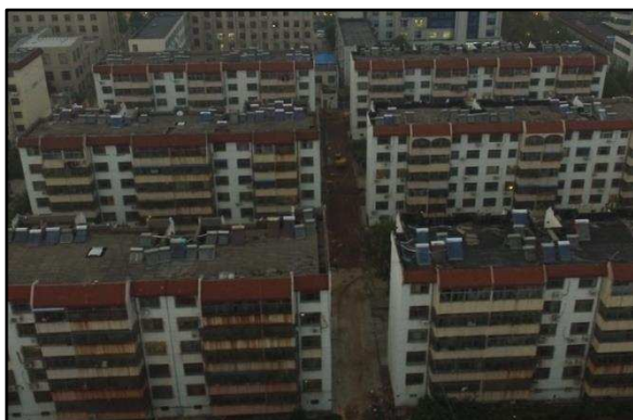
Fig. 5. Individually installed SWHs on the roof of residential buildings in Rizhao. (Photo taken by the first author, 2016)
