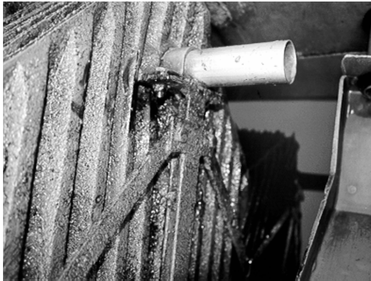
Figure 44 'U' shaped straps clamping the media support through rods to the support frame
