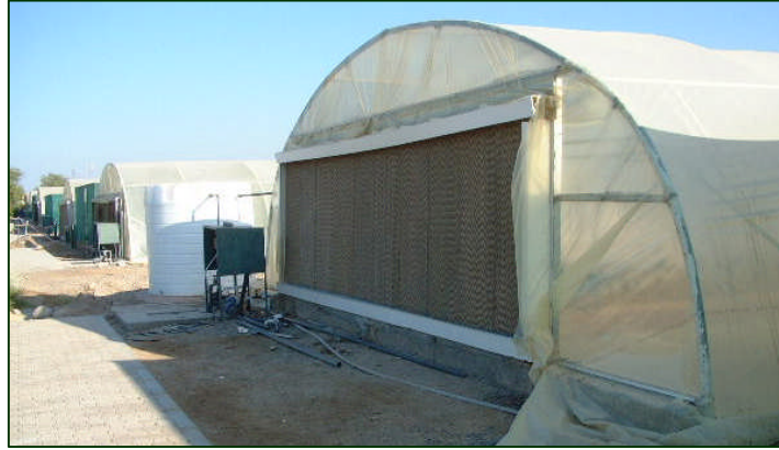
Fig. 2.2: Evaporative cooling pads (i.e. humidifier) at one side of a Quonset greenhouse
