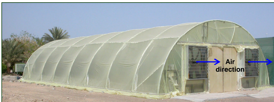
Fig. 2.1: The fans of a Quonset greenhouse
