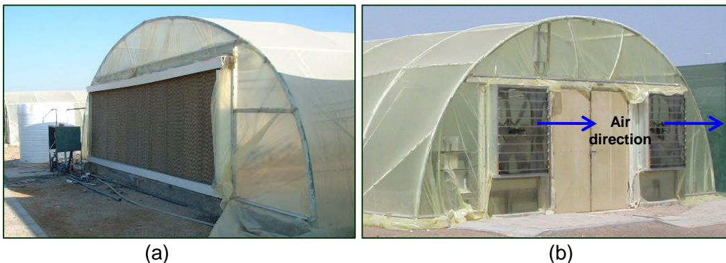
Fig. A1.2: (a) The set of evaporative cooling pads at one side of the greenhouse and (b) the fans at the opposite side
