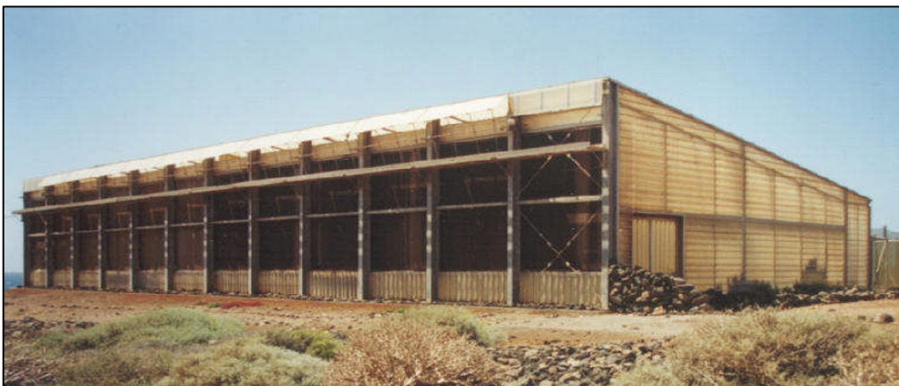
Fig. 2.4: The seawater HD greenhouse in Tenerife (Davies et al., 2004)
