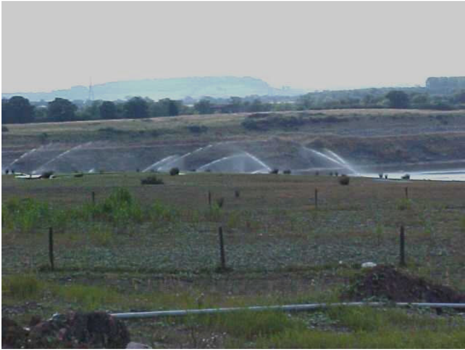
16 Fig. 1. Representative spray irrigation of landfill leachate using spray guns 17 and illustrating typical spray radii
