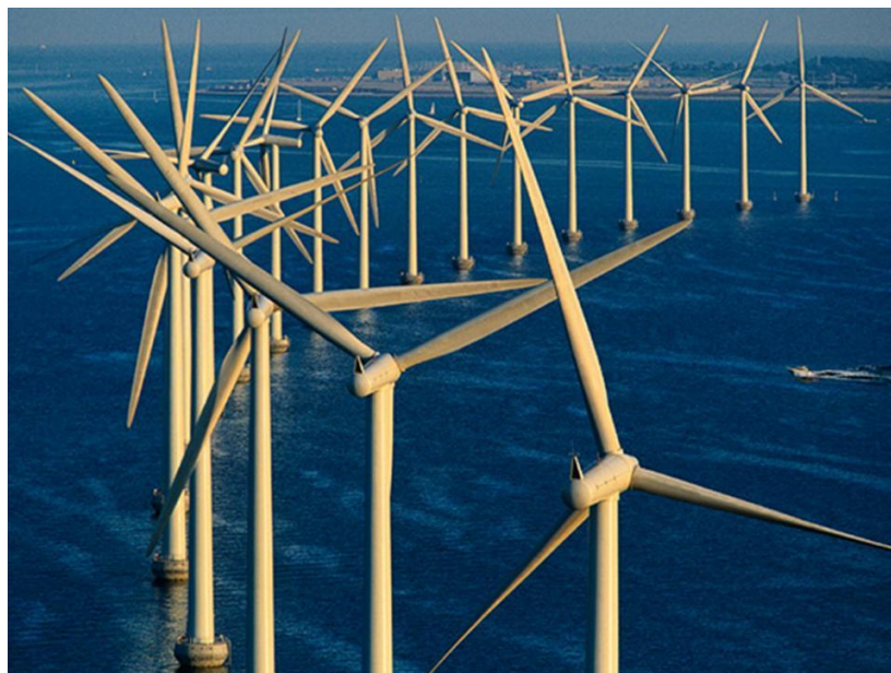
Fig.1 – Example of installations.
