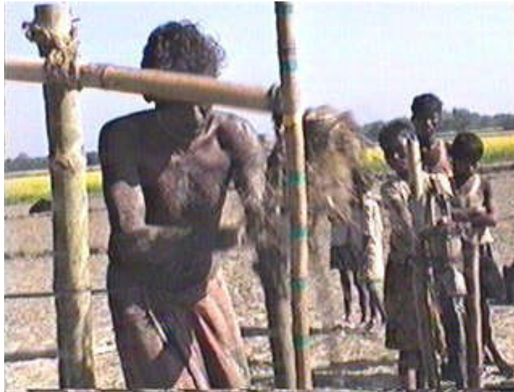
Figure 2: Sludge Ejecting from the Pipe
