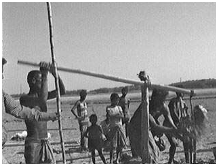
Figure 1: Mistries Operating Sludging Equipment
