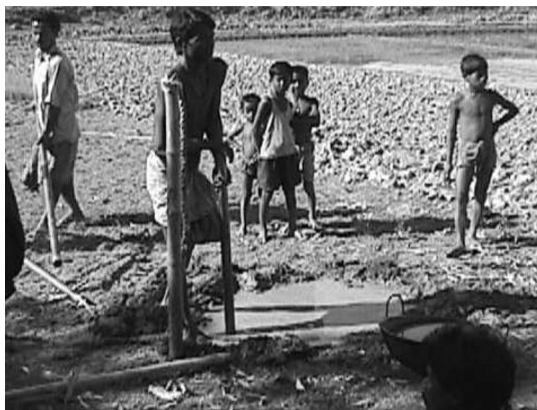
Figure 4: Mistry Starting a Hole with 1.5m Pipe
