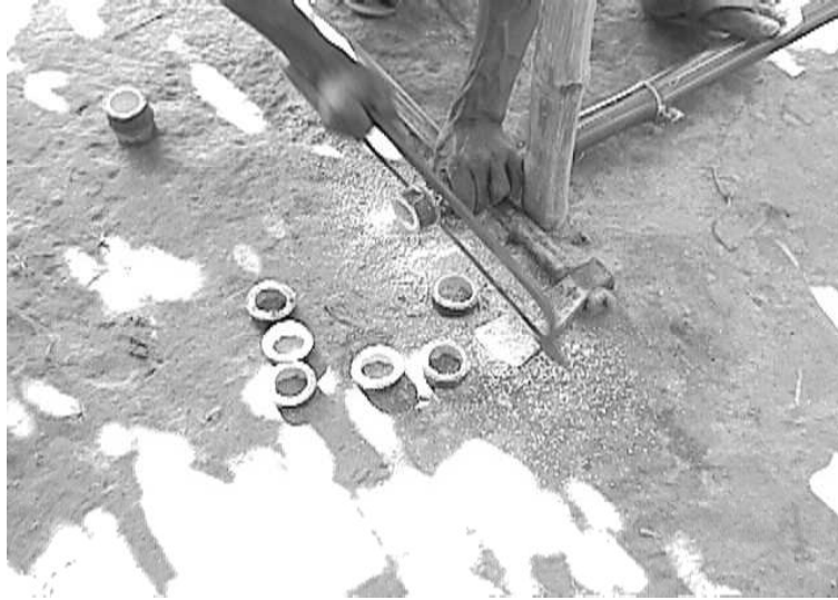
Figure 12: Cutting the Bamboo “Doughnuts”
