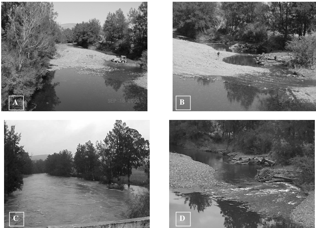
Figure 4: (A) Upper section of Munni test reach at the commencement of construction of DFJ1. Note a 4 m high actively eroding bank was located to the right of the tractor; (B) DFJ1 & 2 at the completion of construction; (C) Same view in flood ( 270 \text{ m}^3 \text{sec}^{-1} , 7/05/01) at about 1 m below peak stage; (D) DFJ1 & 2 after the second major flood since construction—note the aggraded bar upstream of first structure and the increased scour around the two structures. The riffle crest in the foreground was raised, we presume due to backwater effects associated with the structures.
