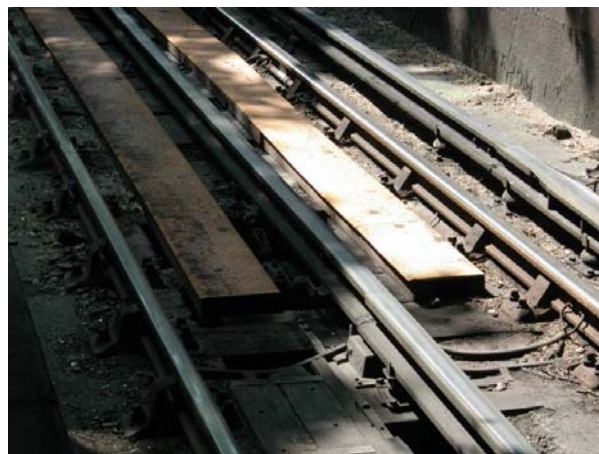
Figure 6-11 Insulated Block Joint
