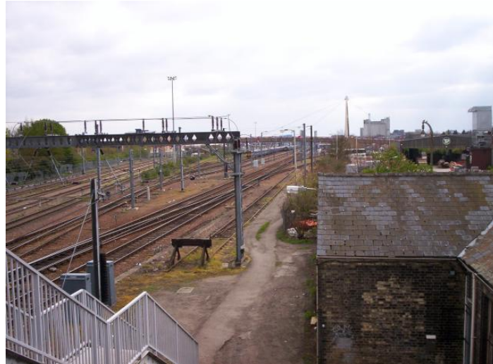
Figure 6-10 Sidings at Cambridge Station
