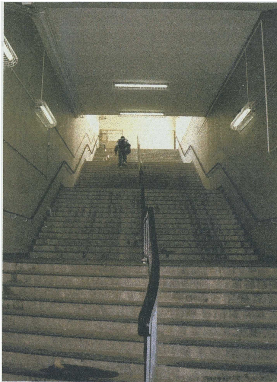
Figure 181 - Looking up the entrance stairs
