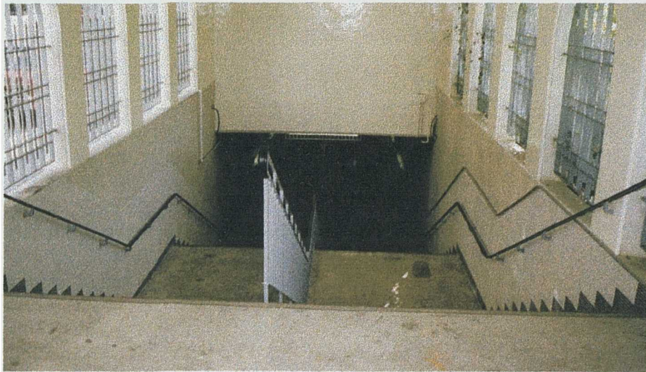
Figure 180 - Looking down the entrance stairs to the infield tunnel.
