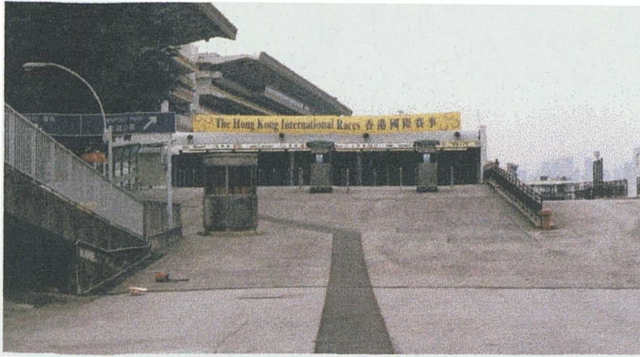
Figure 193 - The approach to gate 1 at Sha-Tin.
