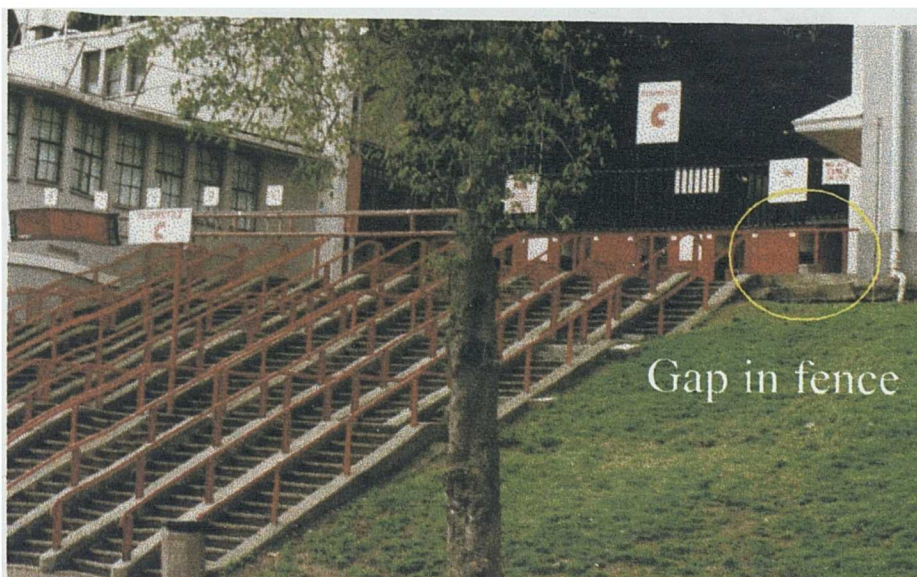
Figure 4 - The gap offers a view of the turnstiles, especially when the stairs are full
