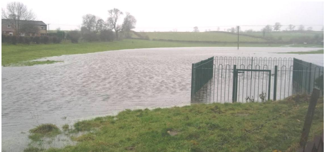
Figure 13 The field behind the properties in Figure 11 and the entrance to the drain (fenced area)
