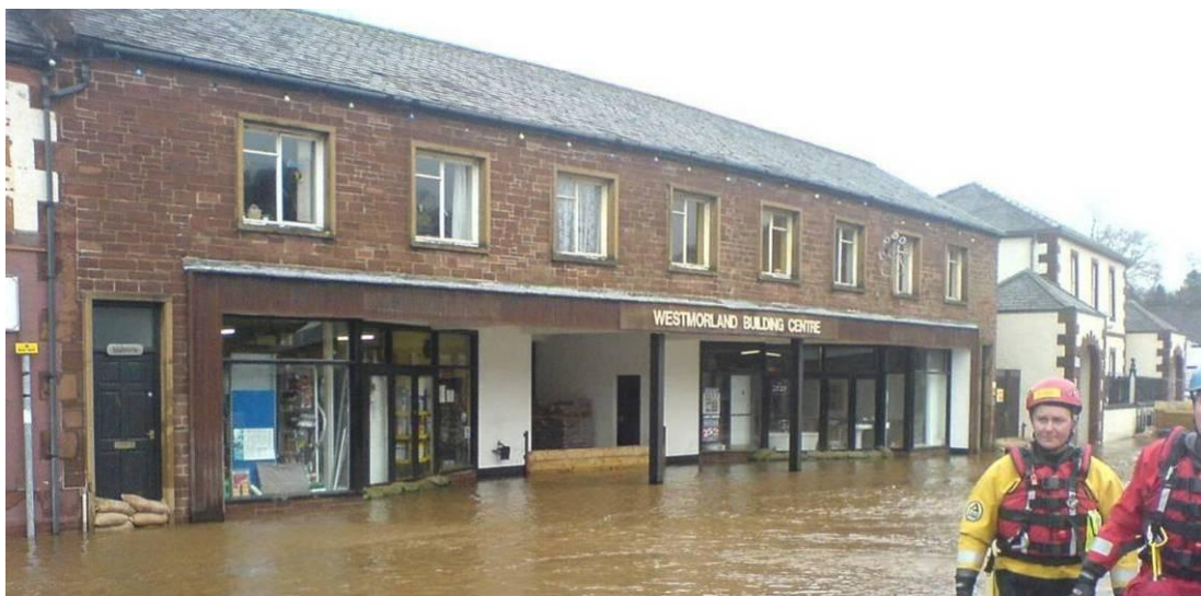
Figure 10 Flood protection measures in action in Appleby before the pilot scheme
