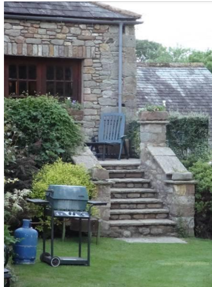
Figure 9 An example of an intrinsic protection measure: a raised building extension
