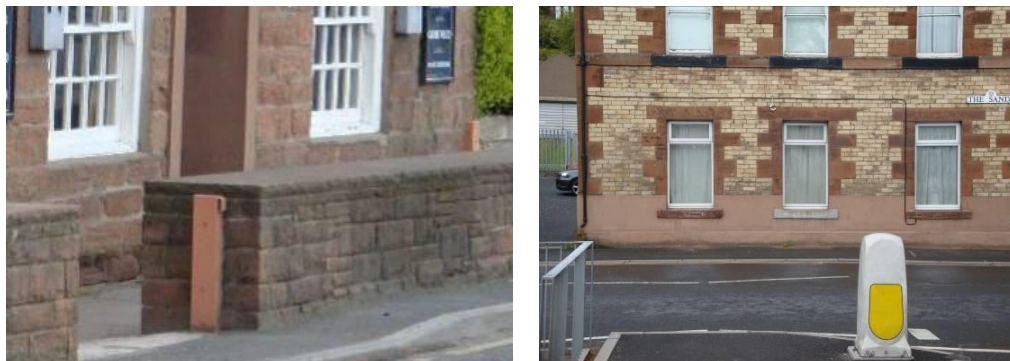
Figure 22 Fixings for deployable barriers (left) and water-resistant render (right)
