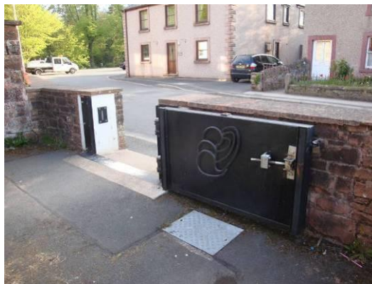
Figure 5 An Environment Agency flood barrier by playing fields in the south of Appleby
