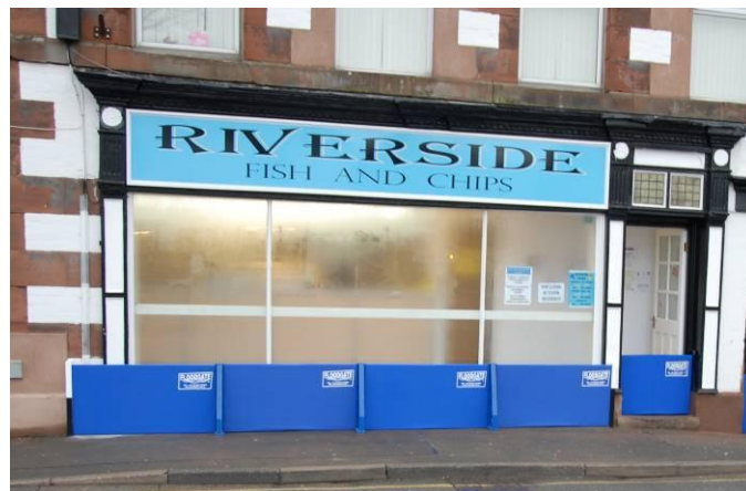
Figure 17 Deployment of barriers in front of a food outlet on The Sands
