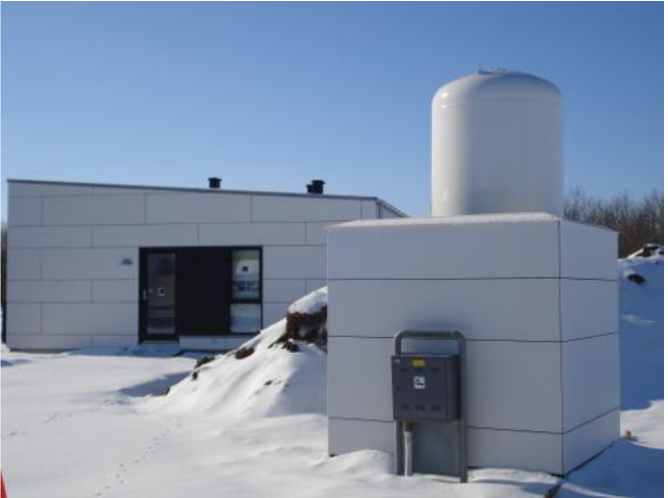
Image 1: Electrolyser building at H2 college
