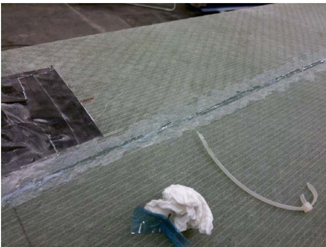
Figure 2. Close up on the bonded and smoothed out adhesive over the fibre
