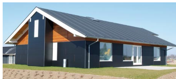
Figure 9: Highly insulated and airtight low-energy house in Kolding (Seest). The house has a mechanical ventilation system with highly efficient heat recovery.
