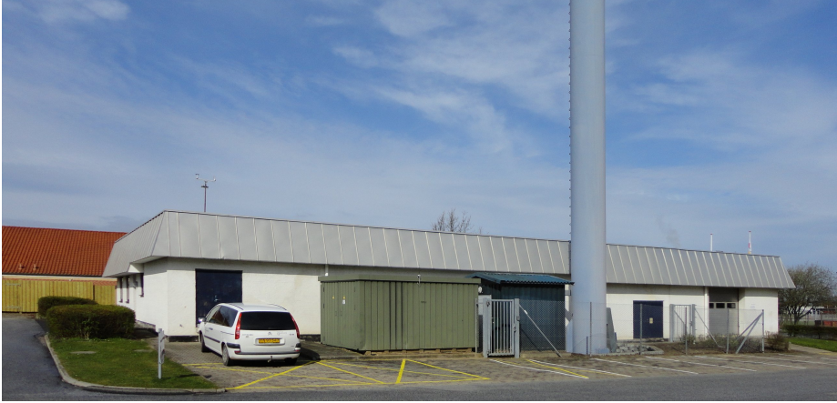
Figure A.1: The weather station in Sønderborg, which is mounted on a pole on the roof of a single-storey district heating plant building (in the image it is on the left side of the building).
