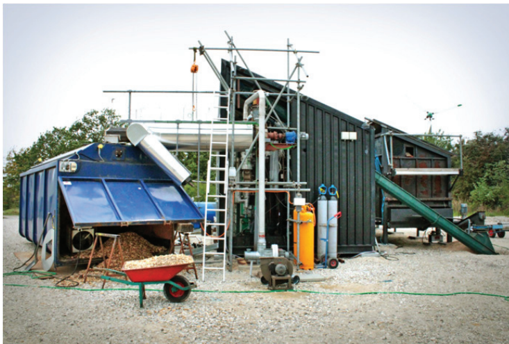
Figure 26: Picture of the torrefaction unit in DTU Risø campus.
