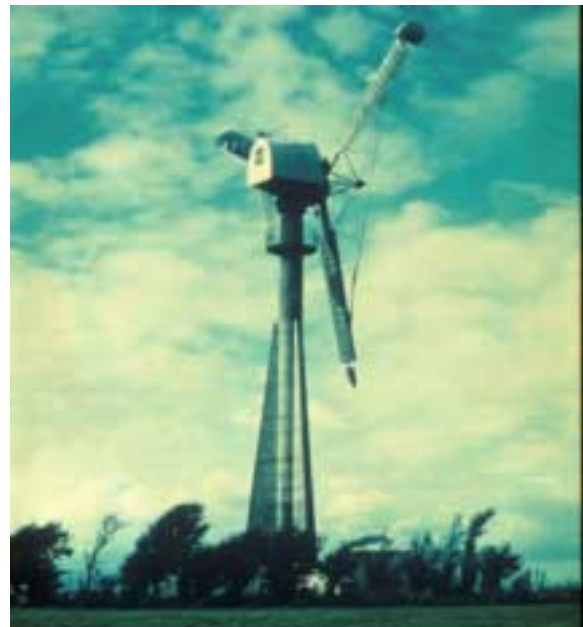
Figure 5 The 200kW Gedser wind turbine, operated successfully from 1956 by the utility SEAS for 10 years
