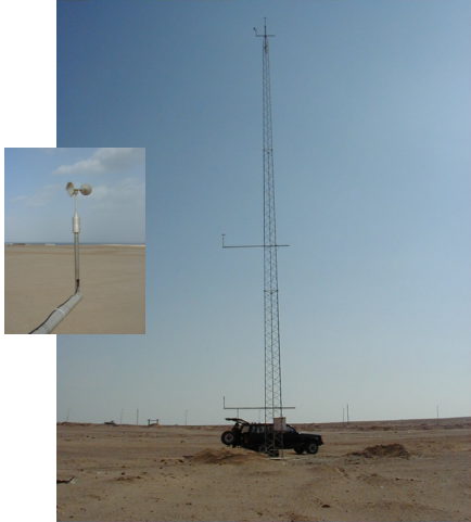
25-m lattice tower, concrete foundation
