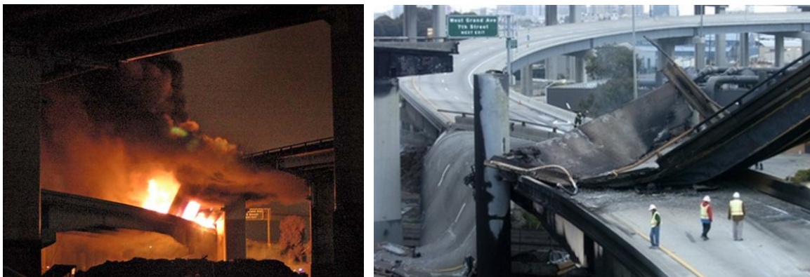
Figura 15. Collasso del San Francisco-Oakland Bay Bridge, ( http://www.sfgate.com/ )
