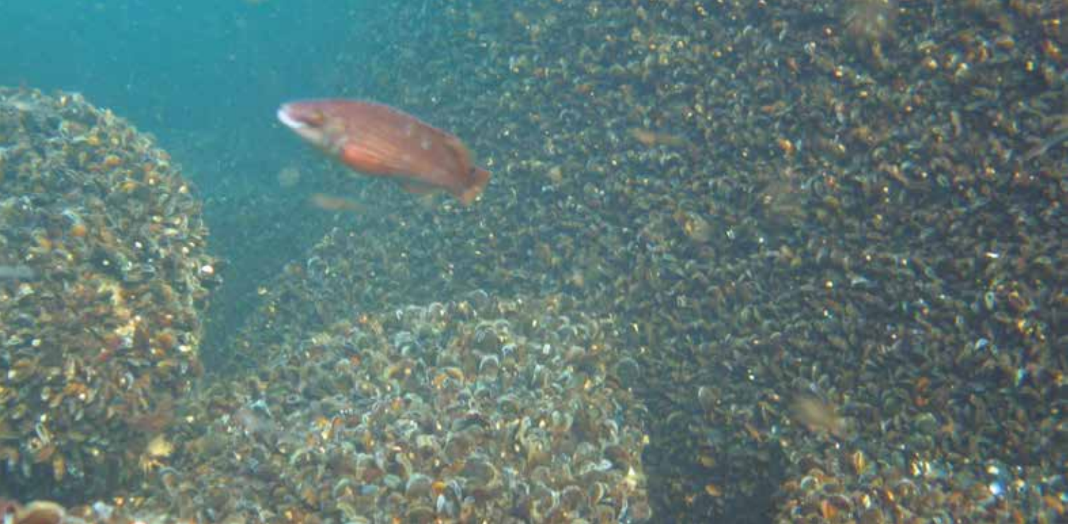
Scour protection with common mussels and foraging goldsinny wrasse at Nysted. PHOTO: MAKS KLAUSTRUP
