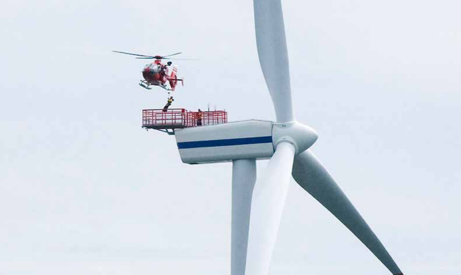
Helicopter servicing turbine at Horns Rev Offshore Wind Farm. PHOTO: VATTENFALL
