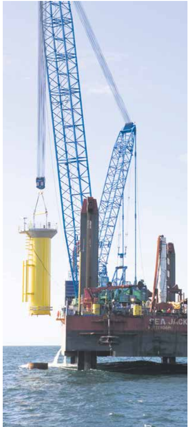
Construction of monopile foundations at Horns Rev 2.
