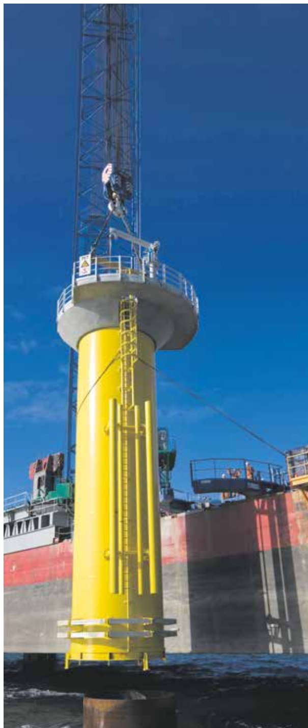
Preparation of monopile foundation at Horns Rev 2.
