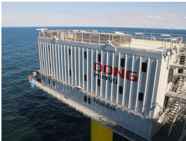
(a) Accommodation platform of the Horns Rev 2 wind farm. A LAWR can be seen on the top left corner of the platform.
