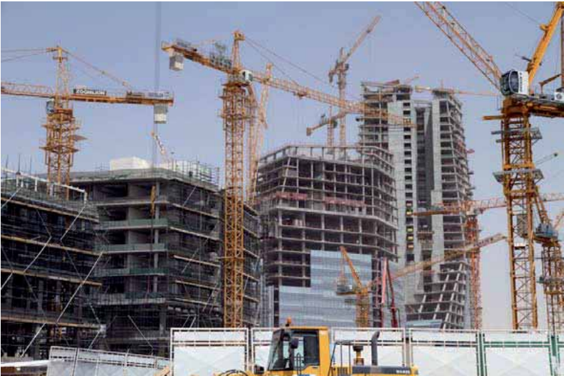
Figure 14: the KAFD construction site in March 2011
