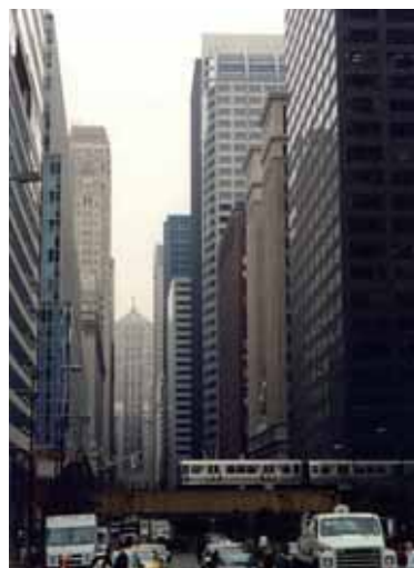
Figure 62: LaSalle Street Canyon. Façade reflectance approximately equal to 15–25%.
