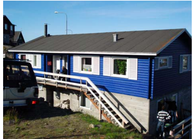
Figure 3: The current view of the blue house with the basement
