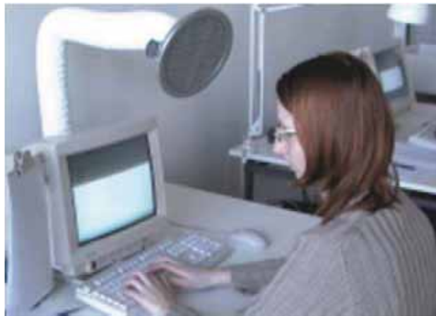
Figure 4.1 Round Movable Panel incorporated in a workstation and used by an occupant.
