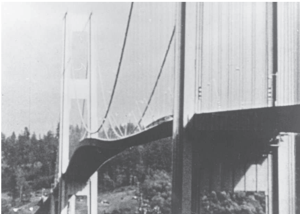
Figure 1.1: The first Tacoma Narrows bridge was strongly influenced by aeroelastic flutter. It collapsed the 1st of July 1940 just four months after opening.
