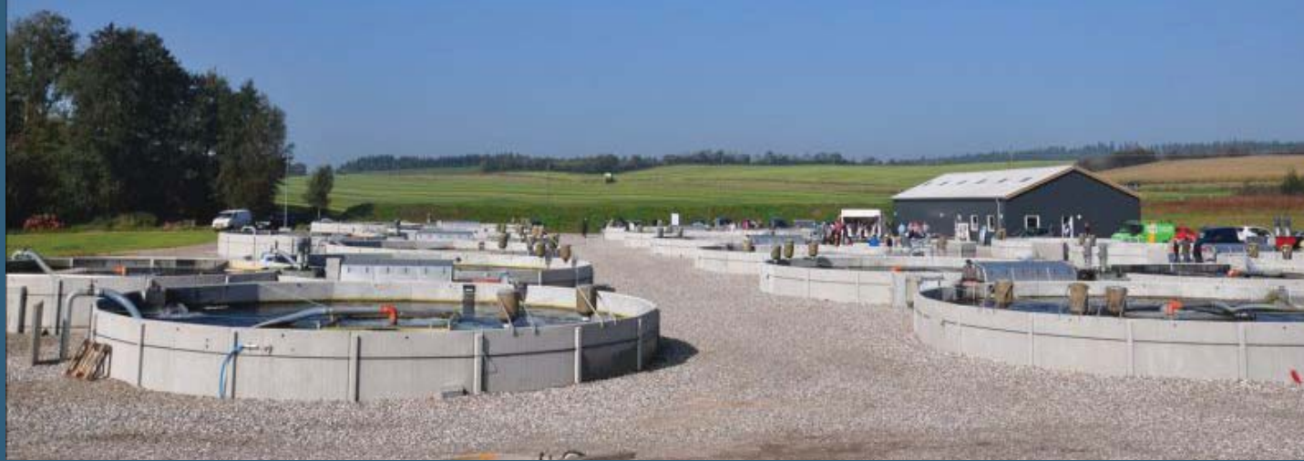
Photo: A freshwater Model-Trout-Farm (Lerkenfeld Fish Farm) which uses circular tanks rather than raceways. (Photo taken by Lisbeth Plesner from Dansk Akvakultur)
