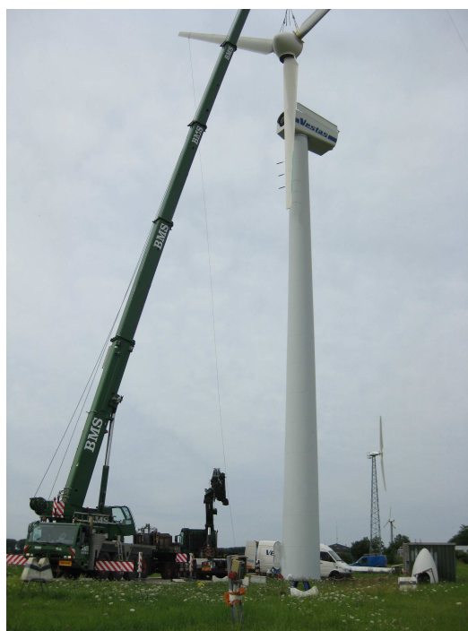
Figure 1. Photo of the V27 wind turbine demonstrator while the rotor with trailing edge flaps is being mounted.
