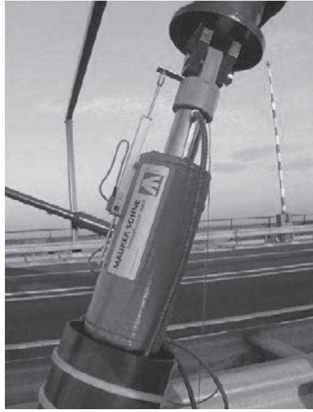
FIGURE 1.1: A Cylindrical Type Magnetorheological Damper (Courtesy of Maurer Söhne GmbH).
