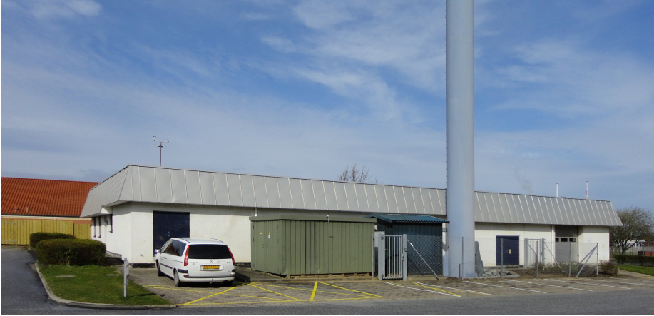
Figure A.1: The weather station in Sønderborg, which is mounted on a pole on the roof of a single-storey district heating plant building (in the image it is on the left side of the building).
