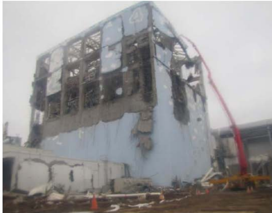
Photo: Water spray into the SFP in Unit 4 using concrete pump truck
