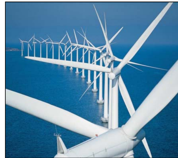
Wind turbine blades made of glass/polyester composites
