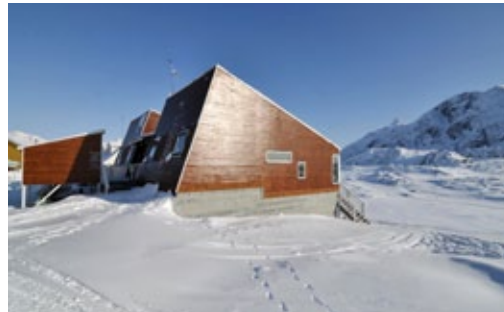
The Low Energy House by Destination Arctic Circle 20
