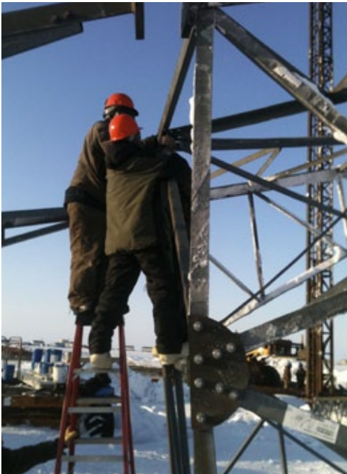
▼ Community members installing wind turbine towers
