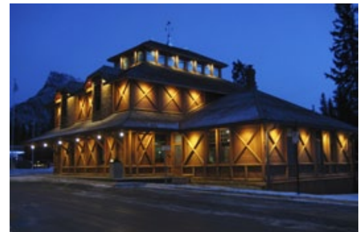
Banff Park Museum lit with low-energy LED lights 14
