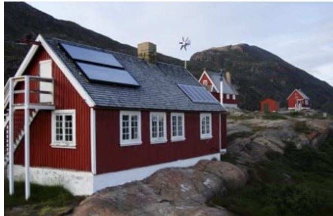
The stand-alone home energy system in Assaqaq, Greenland 5
