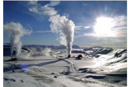
Geothermal power station in Iceland 6
