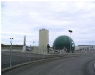
▲ The Biogas storage tank
