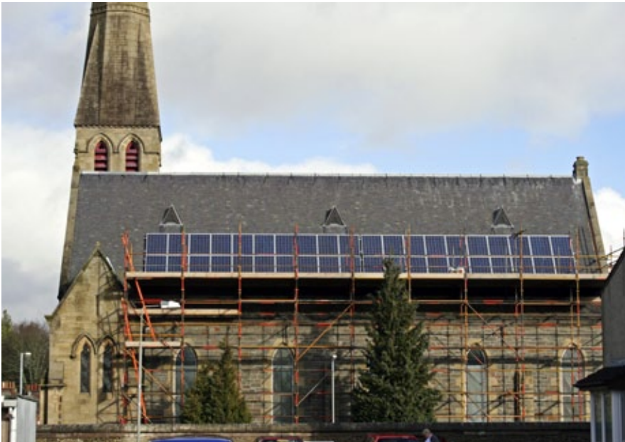
Solar panel installation on a church roof 38
