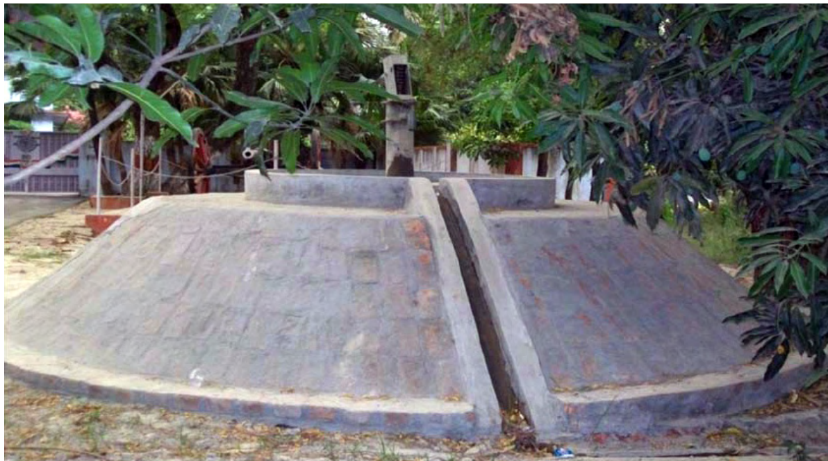
Figure 7: Flood-proofed handpump in Bahraich, Uttar Pradesh, India. The apron is 1-m high, 2.9-m in diameter. The slope of the base is 45-degrees, gradual enough to prevent damage to the base during flash flooding.
