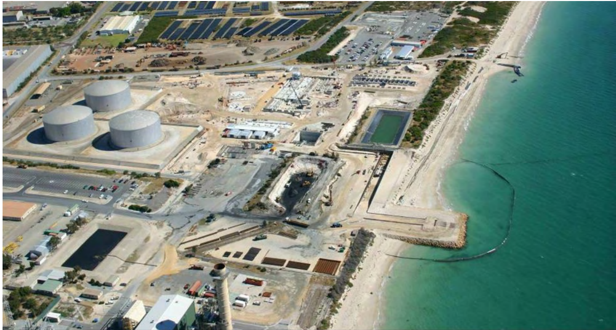
Figure 3: Aerial photo of the Perth Seawater Desalination Plant in Perth, Western Australia. This plant uses reverse osmosis to desalinate seawater.
