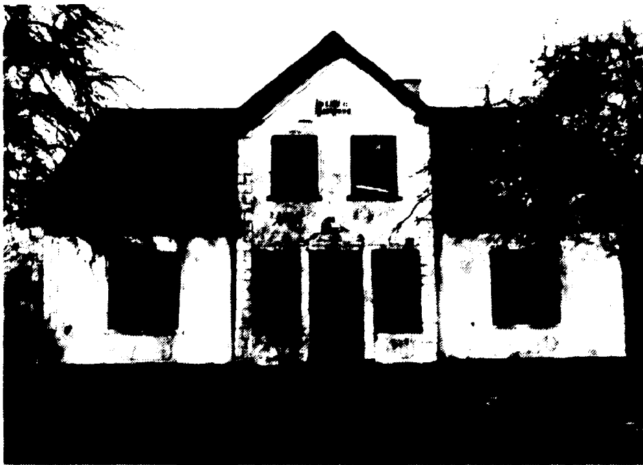
Fig. 3.11.4.2. The farmhouse after 20 explosions.
