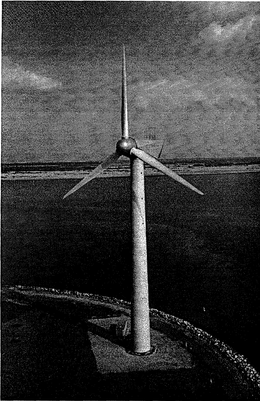
Figure 2-1 The ELKRAFT 1MW wind turbine
