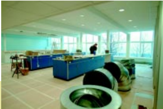
The new pilot plant under construction.
