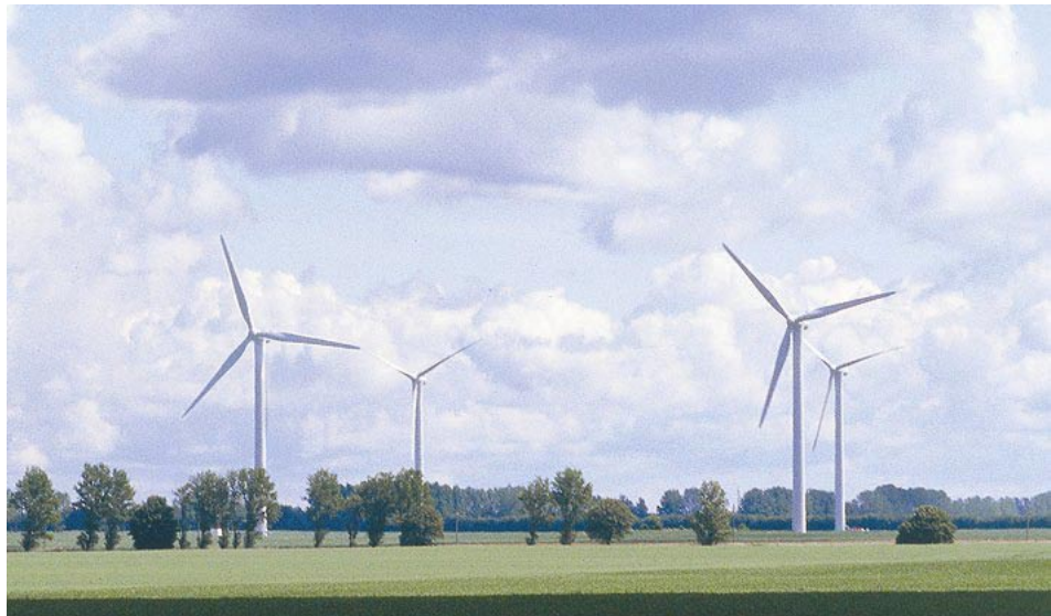
Figure 1. Four of the six wind turbines in Hagesholm wind farm.
