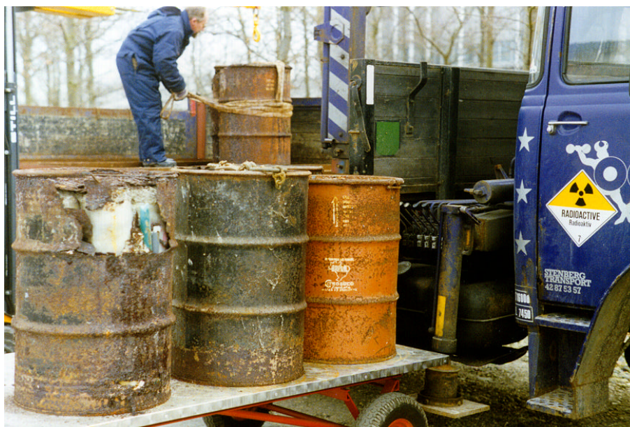
Figure 6.1. Transport of old waste units. The nearest is a badly corroded single layer drum, but in most cases the drums are double: a 100 L drum with the waste material inside a 210 L drum and with the annulus cast with cement mortar.
