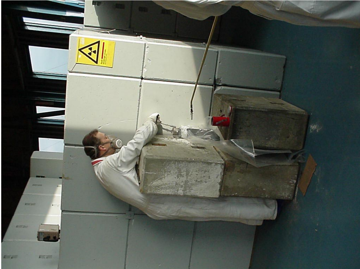
Figure A22. Screws are removed from the top of reflector element No. 60.
