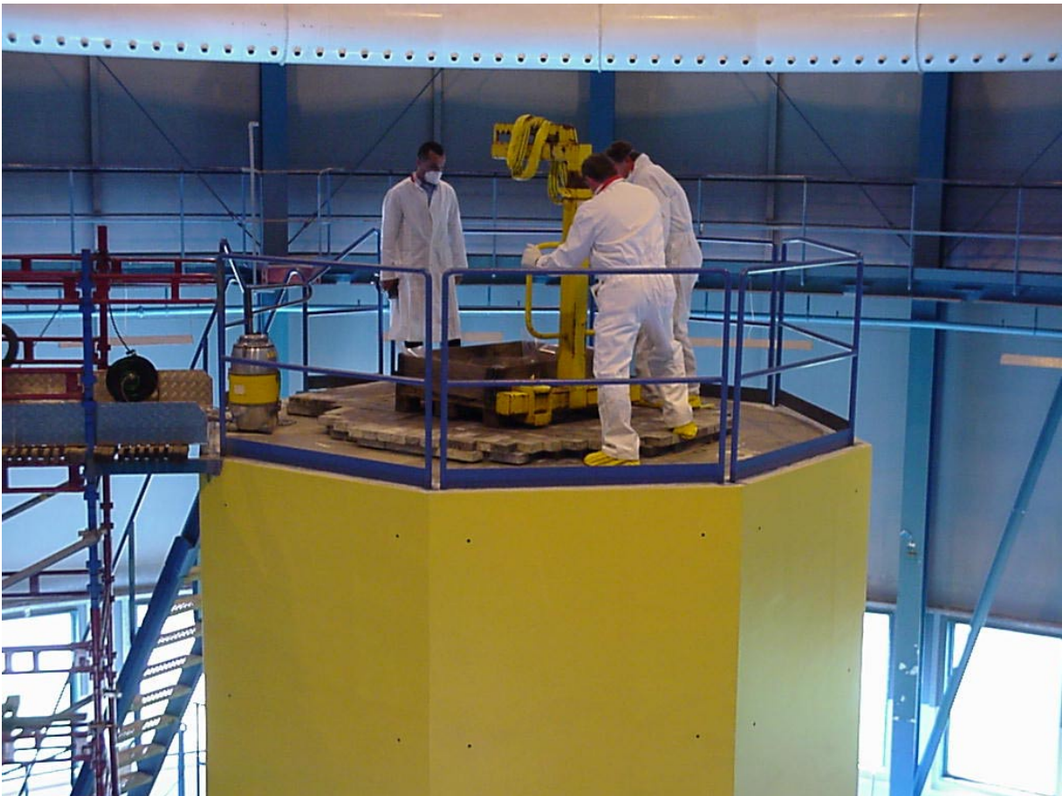
Figure A5. Removal of lead bricks and collection of air samples in the reactor tank.
