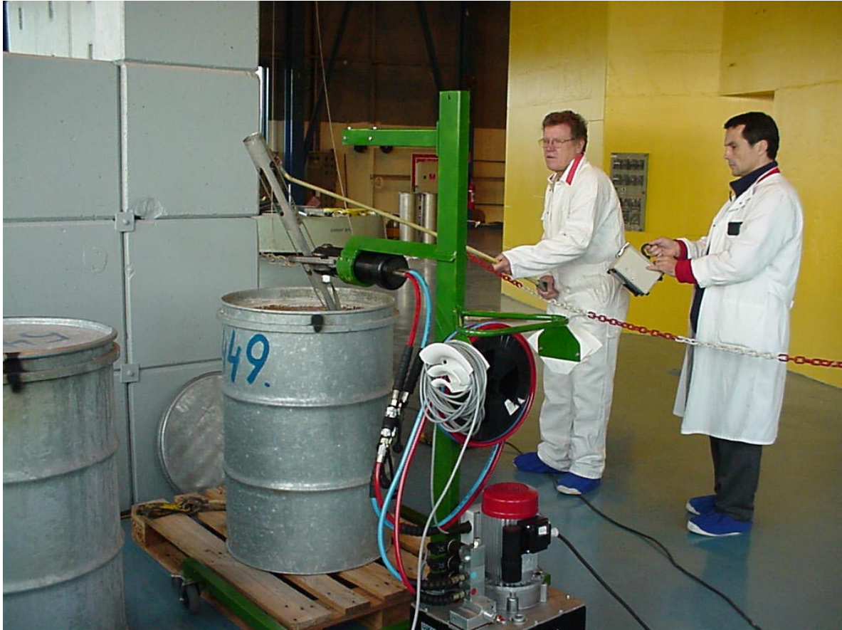
Figure A16. Cutting a guide tube down into a concrete lined waste drum.
