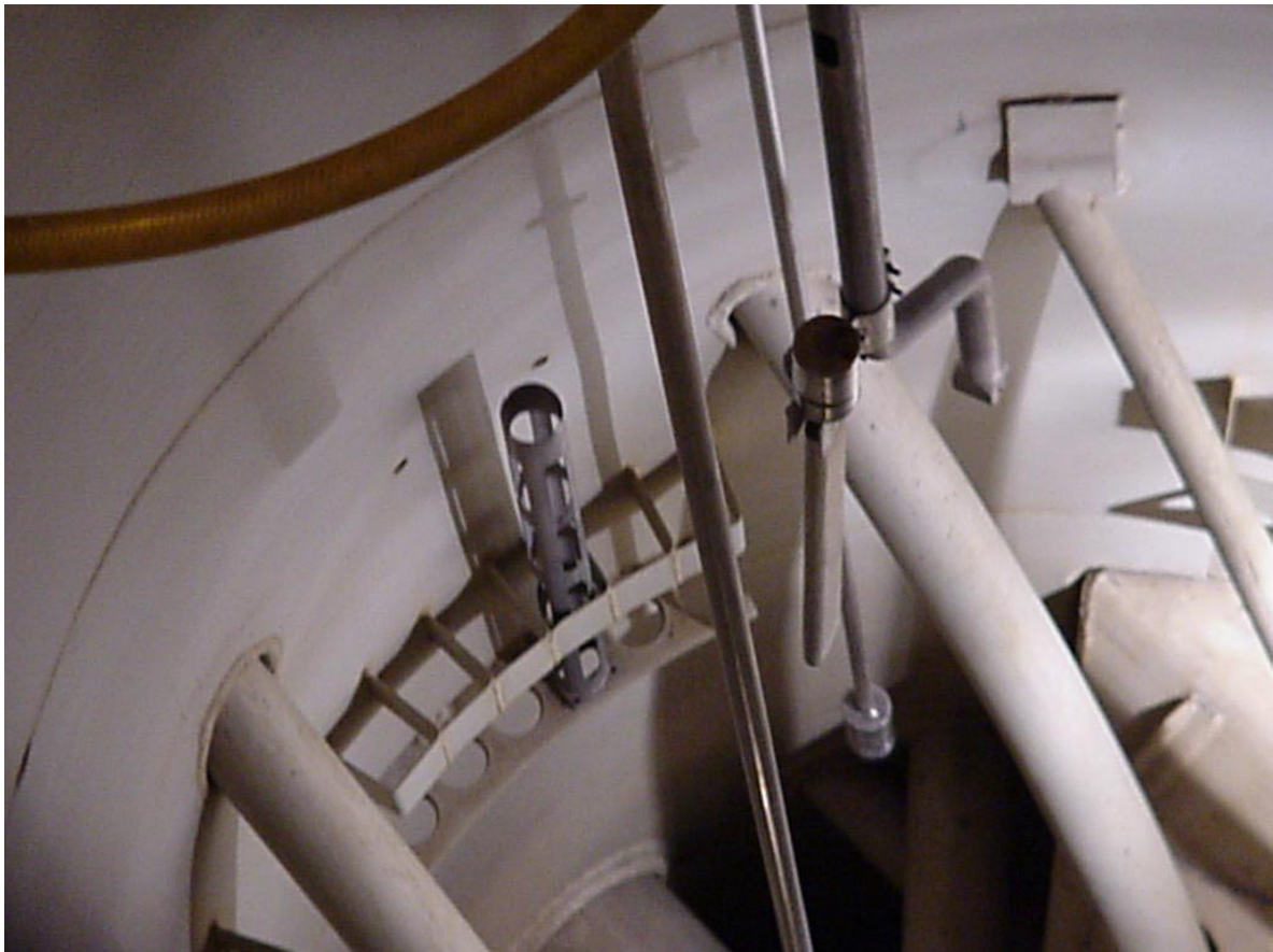
Figure A11. A control rod is lifted out of the reactor tank with the fork shaped tool.
