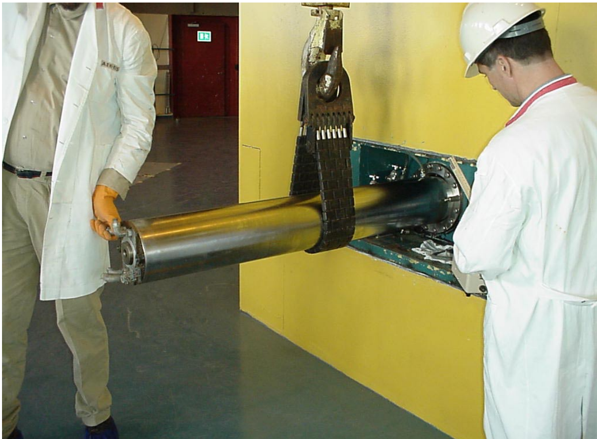
Figure A31. Removal of a beam plug from the reactor block.
