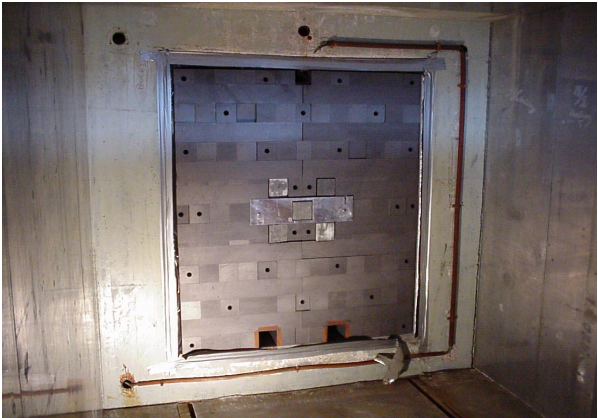
Figure A27. The outer surface of the thermal column in the igloo.
