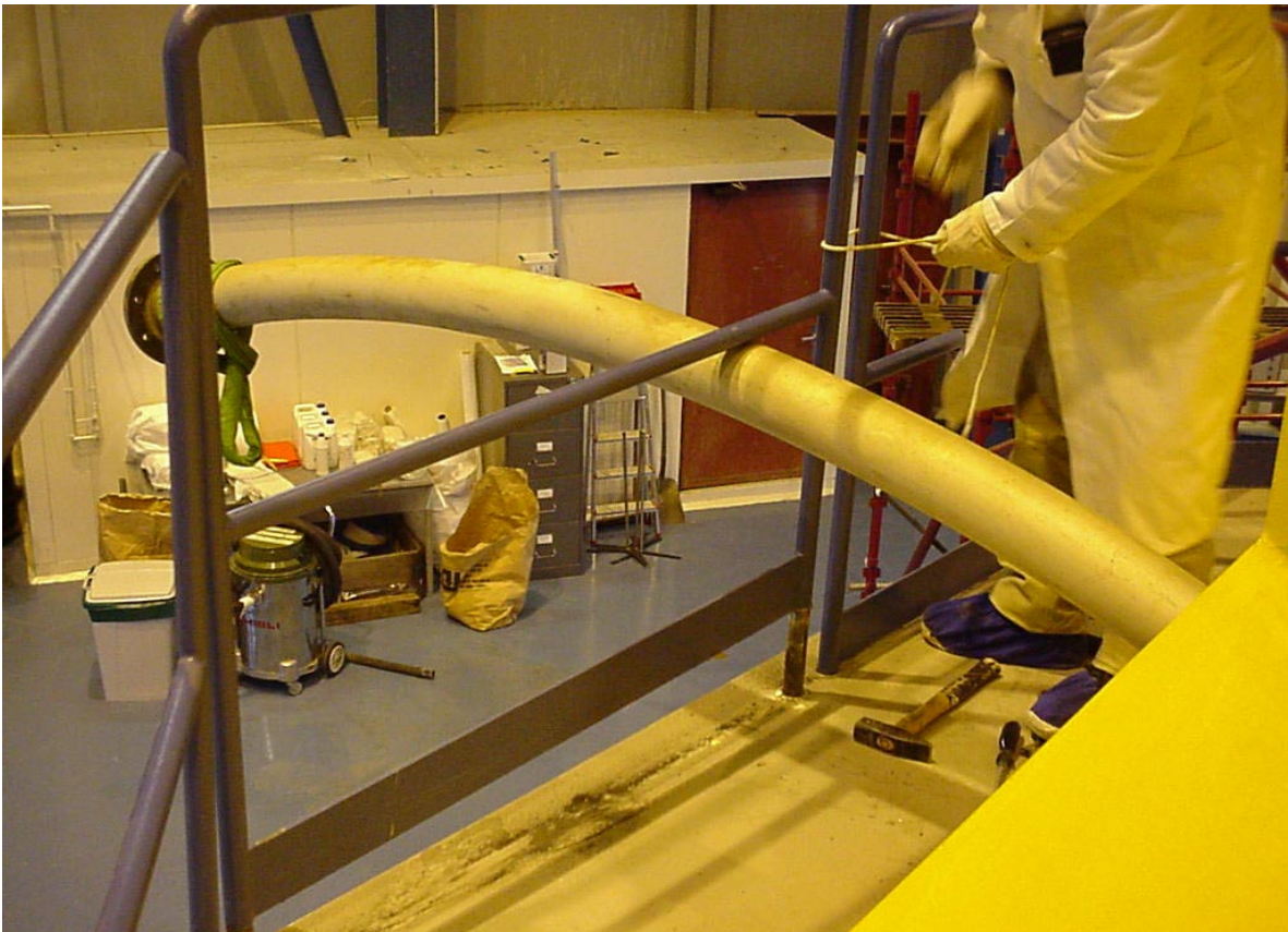
Figure A35. Removal of a S-tube.
