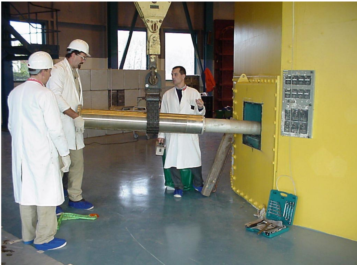
Figure A33. Removal of a beam hole sleeve from the reactor block.
