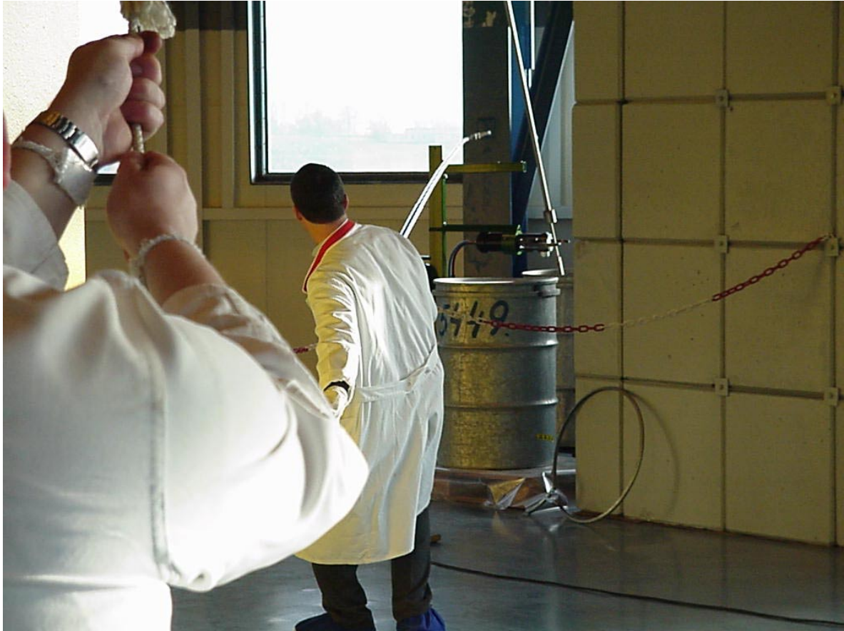
Figure A18. The regulation rod is cut down into a concrete lined drum.
